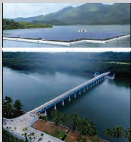
Establishment of 500 kWp Grid Tied Floating Solar Photovoltaic System in Banasura Sagar Reservoir, Wayanad & Construction of salt-water exclusion regulator cum bridge across Kariangode River at Palayi valavu in Kasaragod district.
